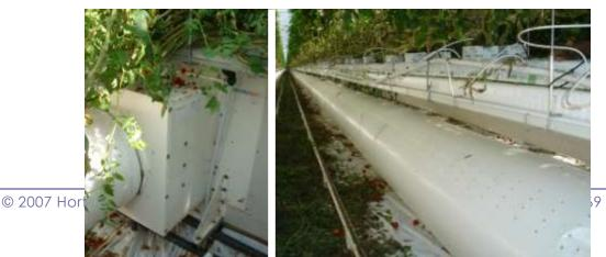
Figure 1 – A ducted Air Treatment Unit
